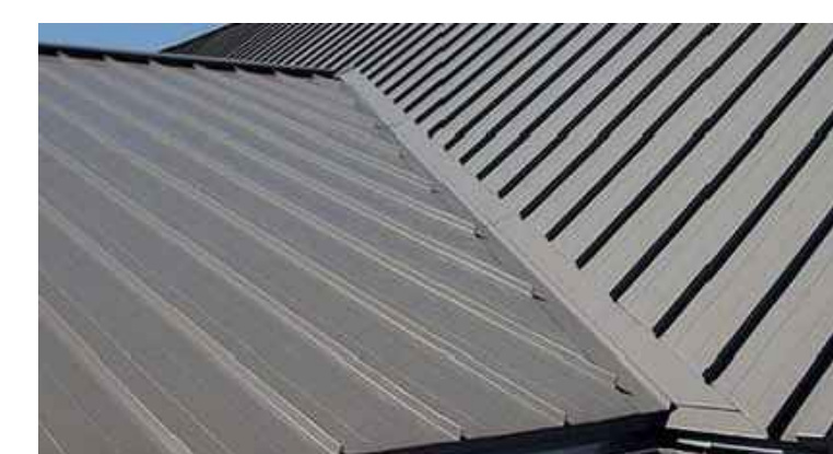
STANDING SEAM METAL ROOF ( MUSTANG GRAY )
