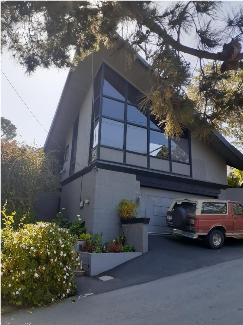
Figure 1: Front elevation looking southeast
