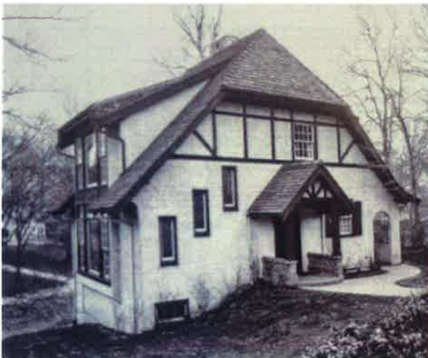
House, Louisville, Kentucky, approx. 1910. Source: McAlester, 2023, p. 456.
