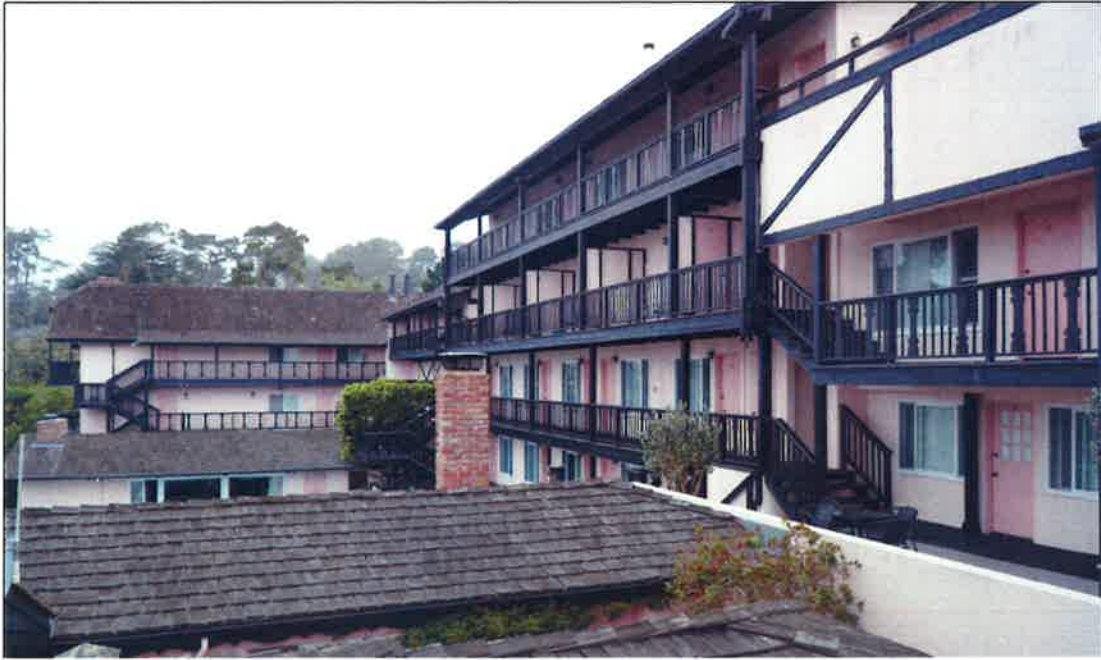
Figure 3. Looking along west side of Hofsas House Hotel, toward north wing, from steps leading to office, 29 July 2022.
