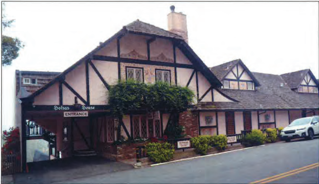
Figure 1. Looking northwest at east side of Hofsas House Hotel, 29 July 2022.
