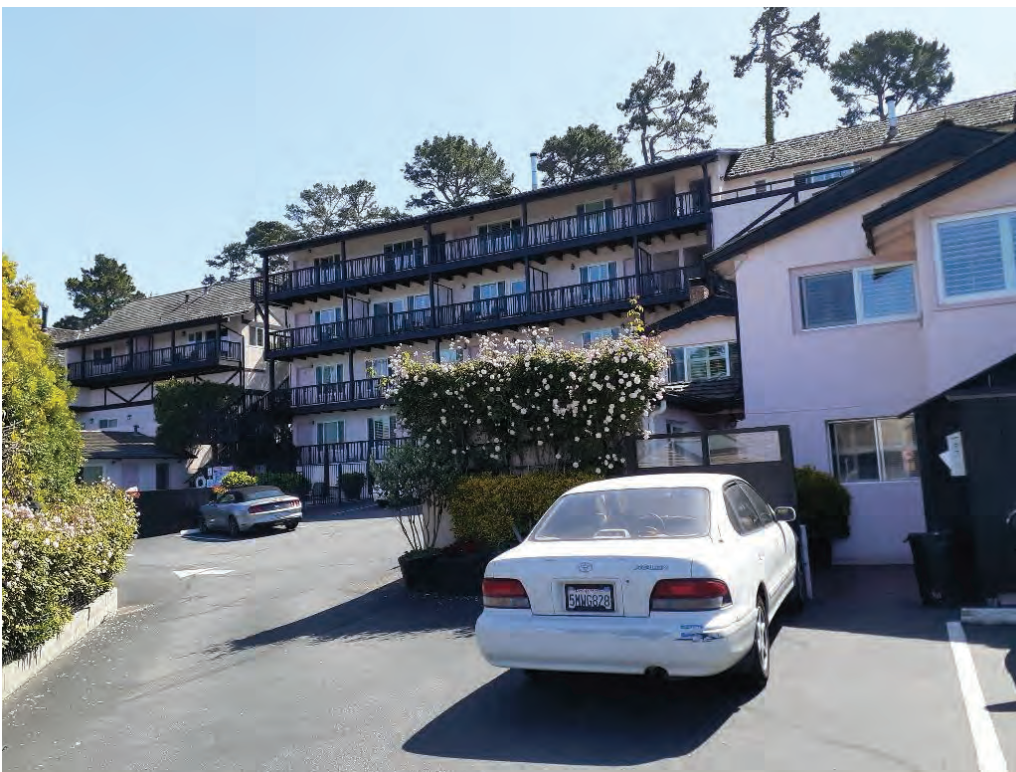
Figure 5: Rear elevation of 1957 hotel looking northeast.
