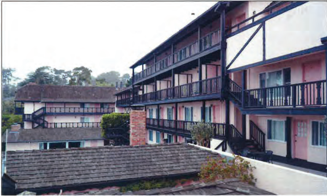
Figure 3. Looking along west side of Hofsas House Hotel, toward north wing, from steps leading to office, 29 July 2022.
