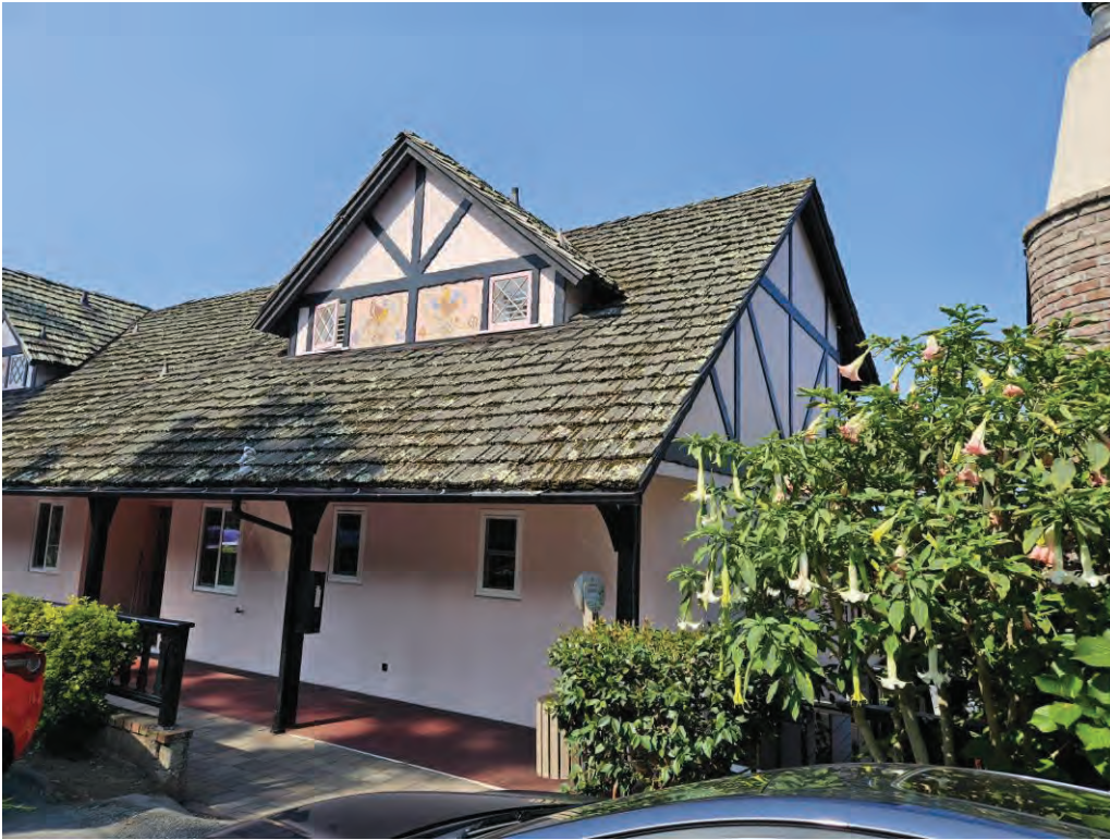
Figure 2: North wing looking southwest from San Carlos Street.
