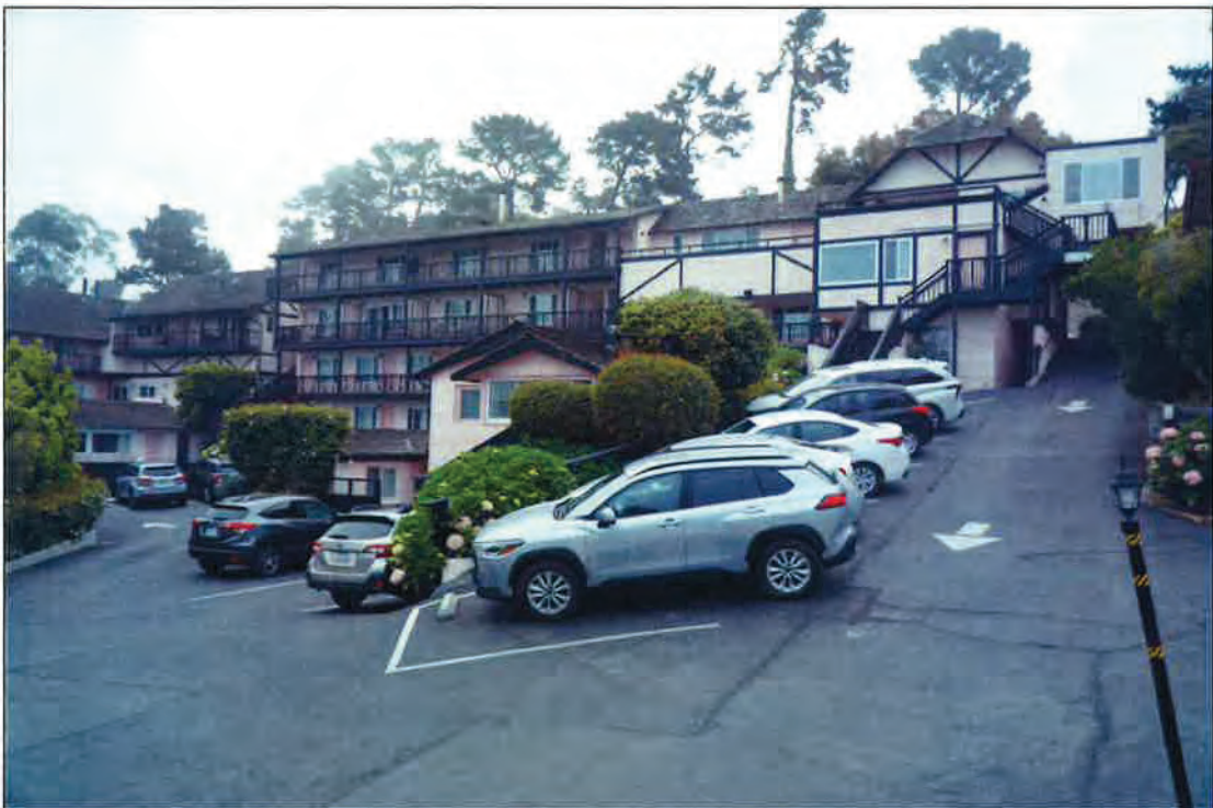
Figure 2. Looking northeast at west side of Hofsas House Hotel, 29 July 2022.
