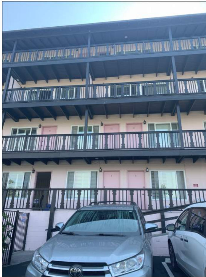
Figure 8- Typical Exposed Framing at Walkway
