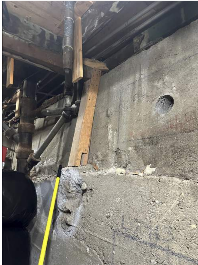
Figure 5- Resupport of 1957 Structure at East Wall of Original Structure
