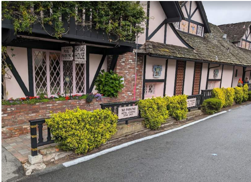
Figure 15 – Existing Pedestrian Loading Zone
