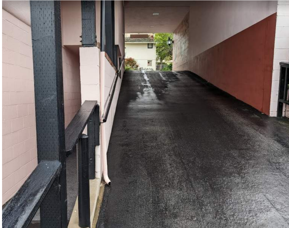
Figure 23 – Ramp at Primary Entrance Driveway
