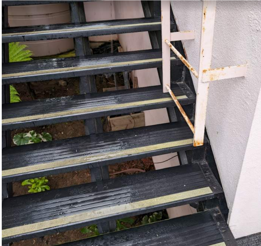
Figure 28 – Gas Meter Under Stairs
