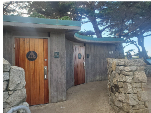
Restroom near Santa Lucia Ave
