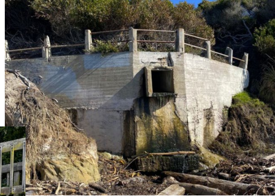
Shoreline: Fourth Avenue Outfall
