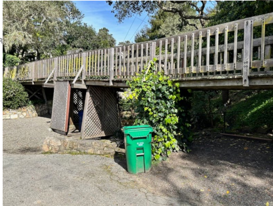
Lincoln/Fourth Trestle Bridge
