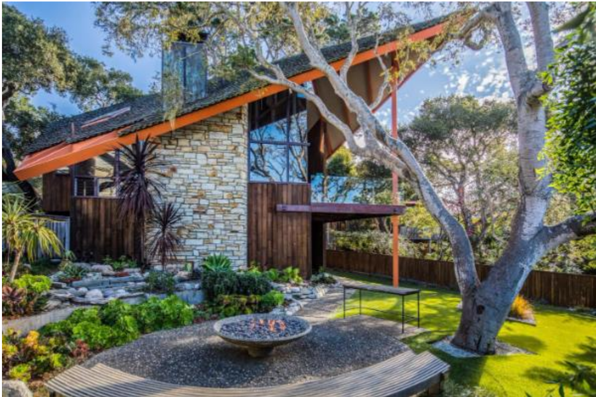
Structural wood post (orange) supporting balcony and roof to be replaced
