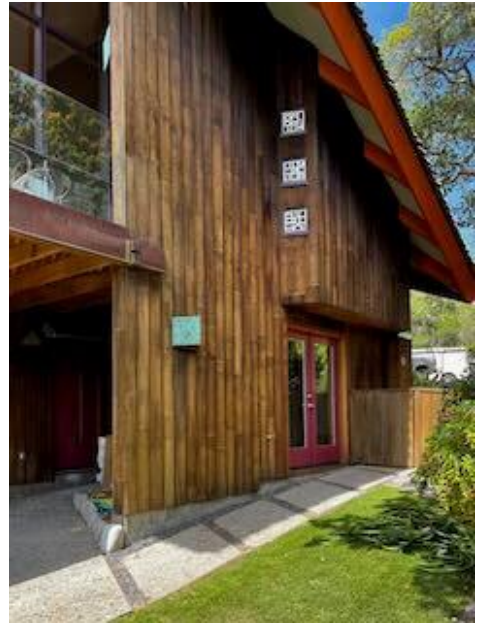
Exterior Redwood Siding and Deck
