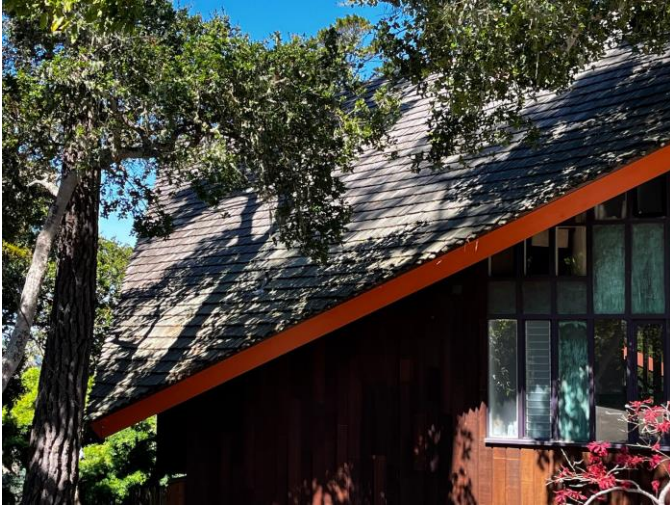
Replace Roof Shakes
