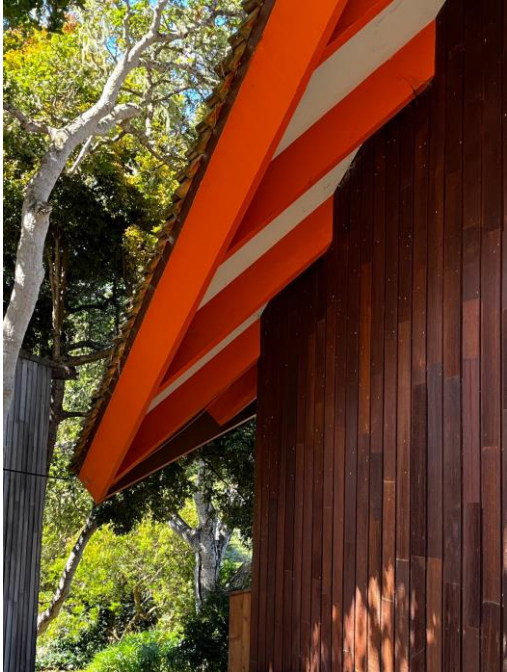
Paint Beams and Ceiling
