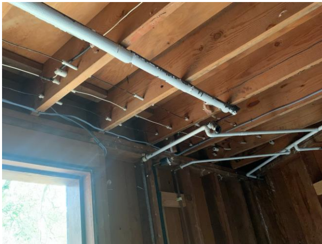
Knob and Tube Wiring
