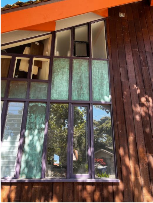
Paint Door and Window Trim
