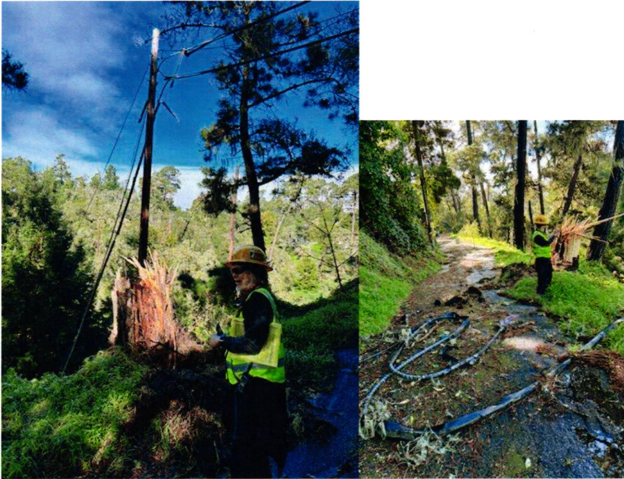
On 2/5 , the lines yanked down from above photos were also connected to CERT volunteers Deanna Dickman & Diana's block on Palou & N. Casanova which caused a jerk on their lines and broke a rotten cross beam on the pole jerking all of the wires. They have sagging wires and no electricity on this block. Photos:
