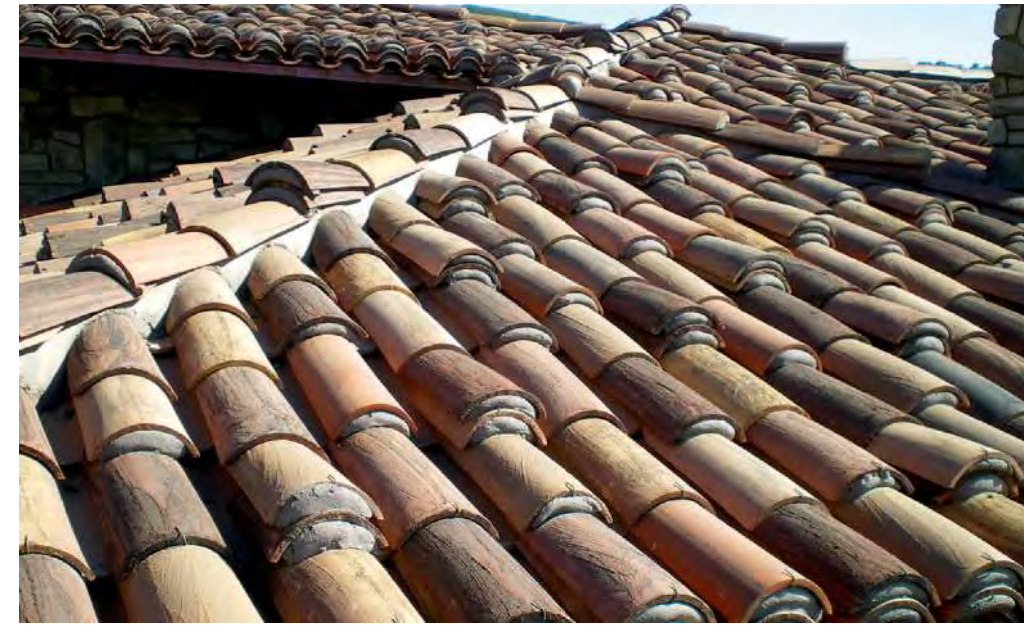
MCA CLASSIC TAPERED MISSION CAP AND PAN CLAY TILE (VINTAGE BUFF COLOR FAMILY, CB-383R TEJA BIANCO BLEND) OR EQUAL
