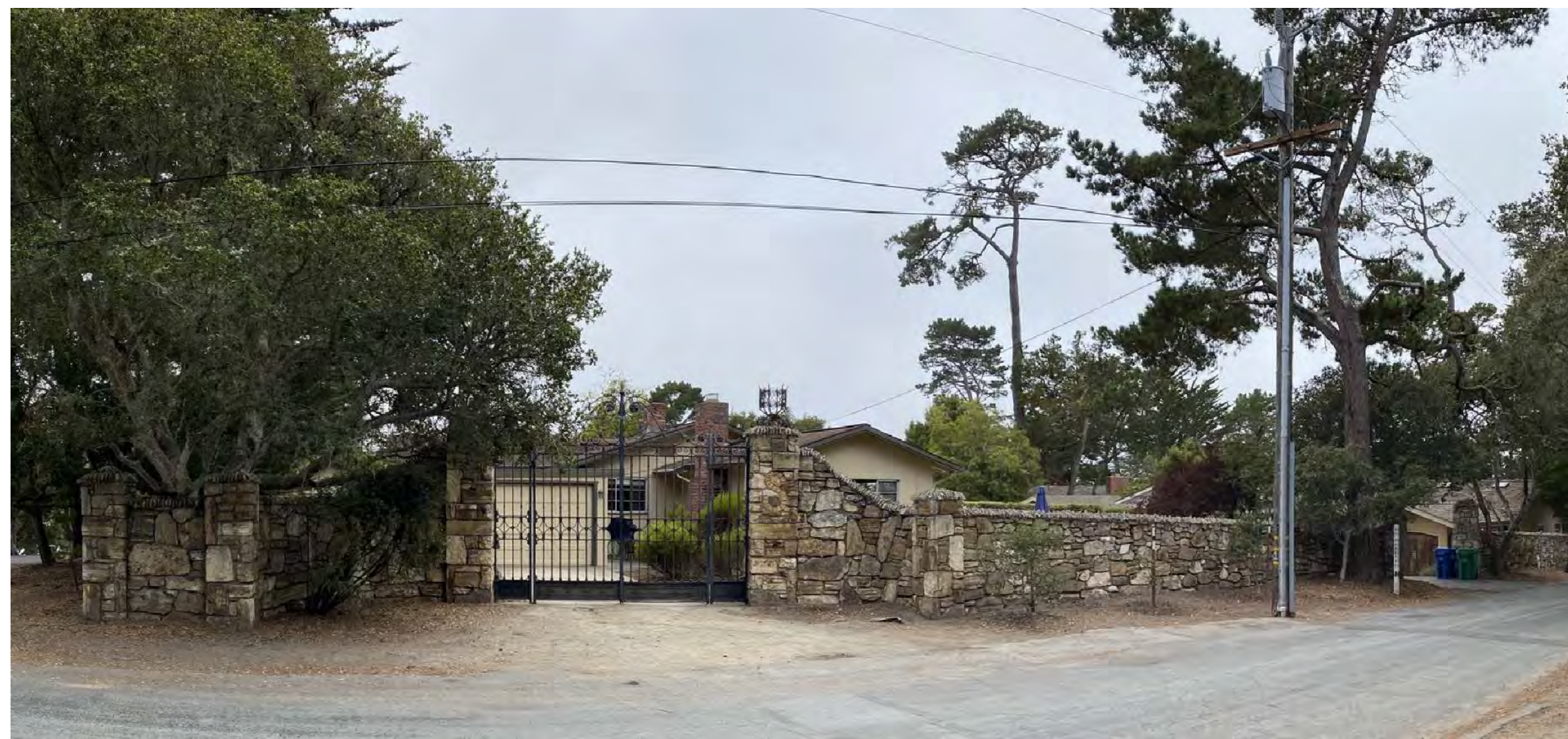
FRONT VIEW BEFORE
