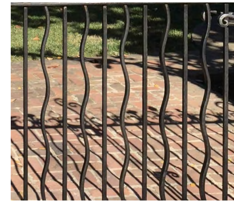
TYPICAL WROUGHT-IRON RAILING.
