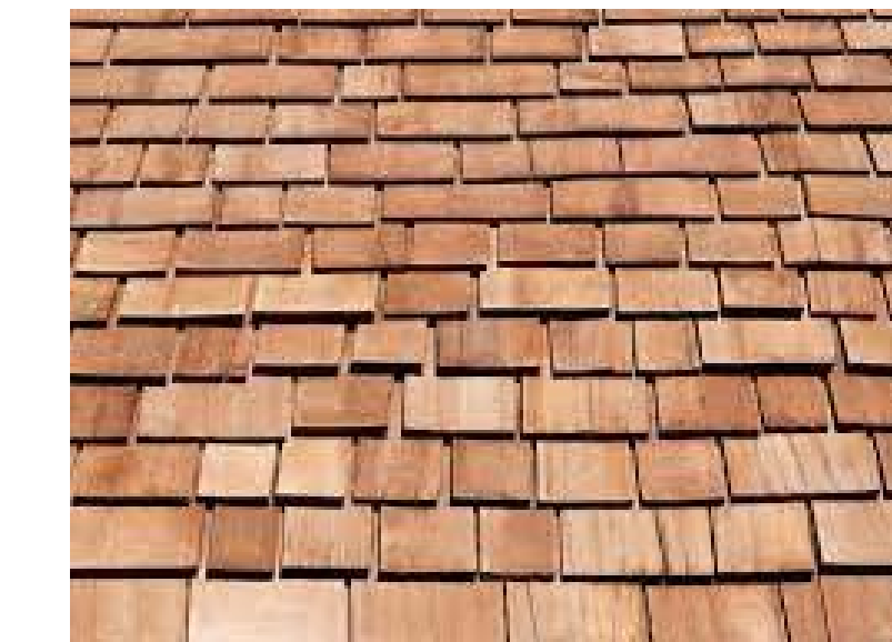
7.18 - FIRE TREATED CEDAR SHINGLES TO MATCH EXISTING
