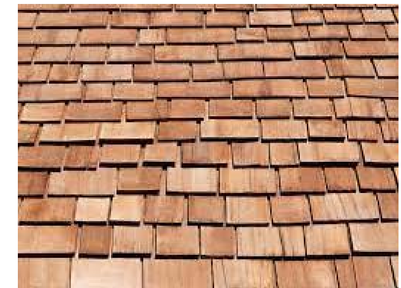
7.18 - FIRE TREATED CEDAR SHINGLES TO MATCH EXISTING
