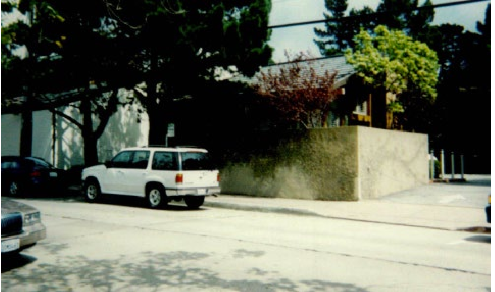
Figure 3b. Photo of original concrete wall submitted as part of application materials for DR 99-35.
