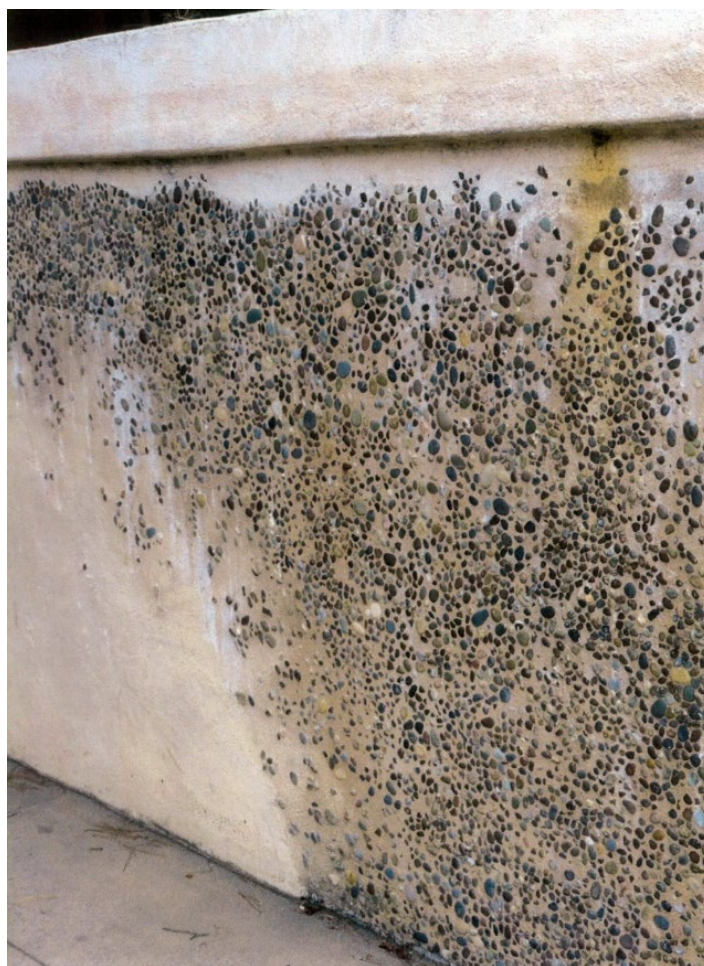
Figure 6b. Photos from application materials submitted with DR 13-24 (Photo 2). Photo is of the mid-section of the wall fronting Dolores Street (see Figure 5, above). Wall has been installed with a planter, a lip has been added to the top area around the planter, and the wall appears to have been partially plastered over. Original aggregate is shown on the right with plastered area shown on the planter lip and left side of the wall.
