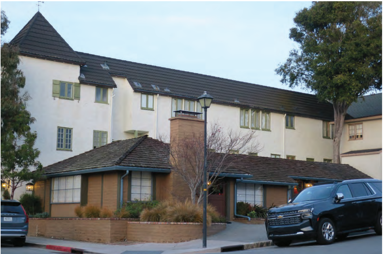
Figure C-21 NE Corner Monte Verde & 7 th Site (Site #20)
