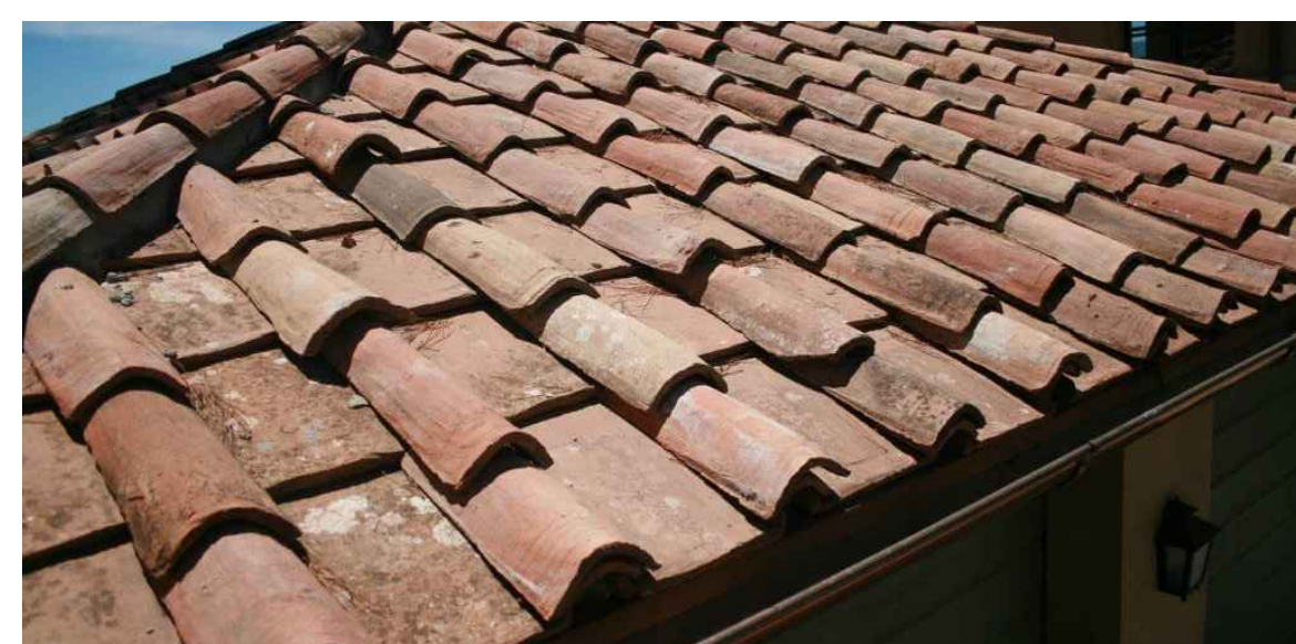
ROMAN STYLE CAP & PAN CLAY TILE ROOF, BUILDING-2
