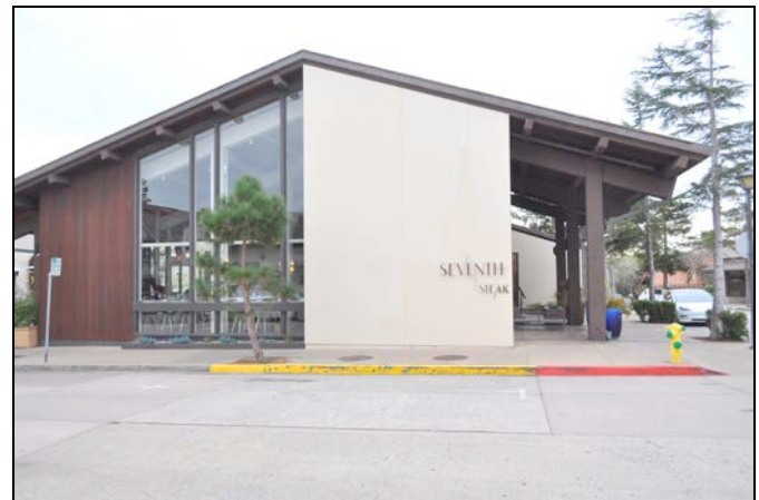
Figure 4. North (7 th Ave.) elevation.
