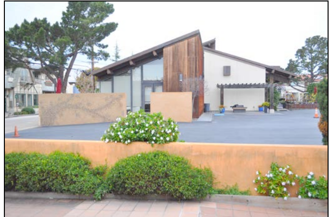
Figure 6. South elevation, with Community Room.
