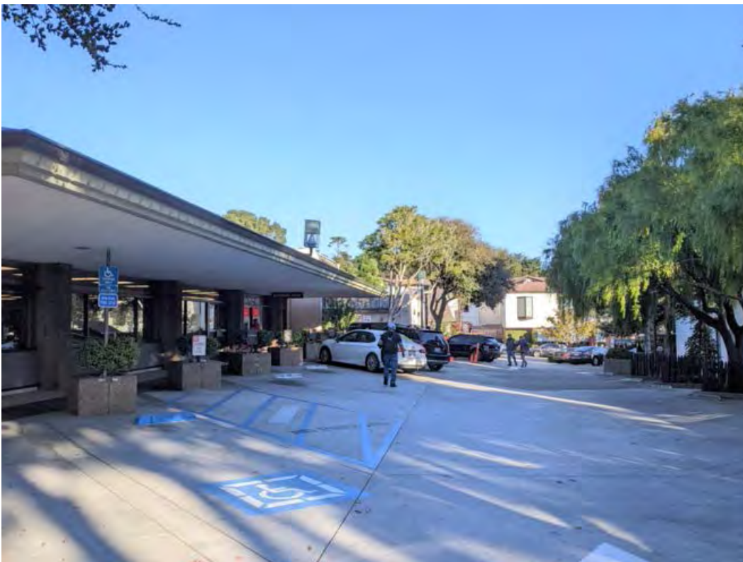
Figure C-12 Wells Fargo Site (Site #11)
