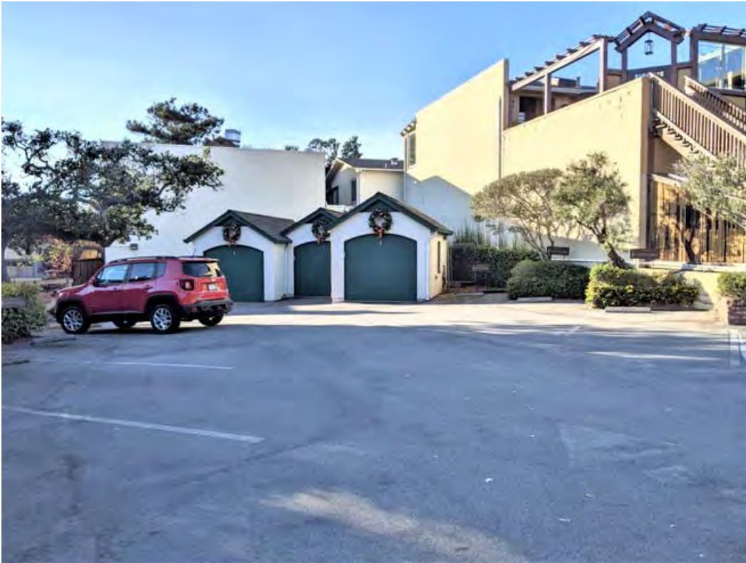
Figure C-8 Three Garages Site (Site #7)
