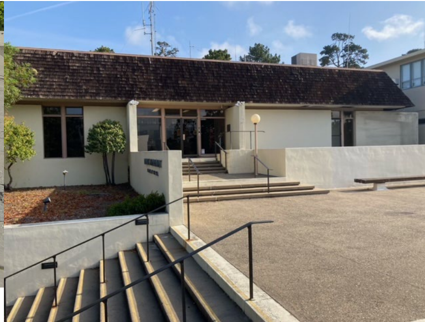
Police Building Renovation
