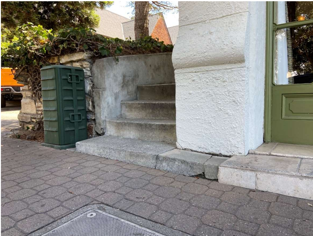
Photo #10, cracked step/foundation at Northwest building corner
