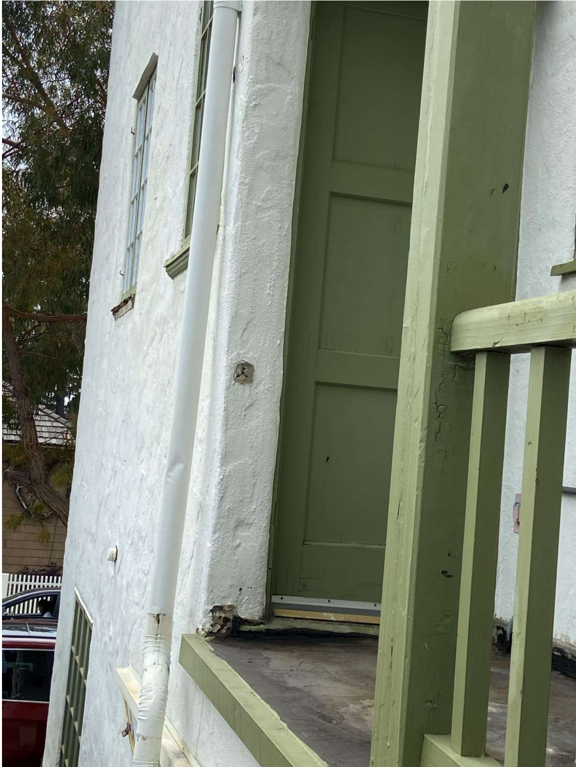
Photo 14, Water damage at upper-level balcony
