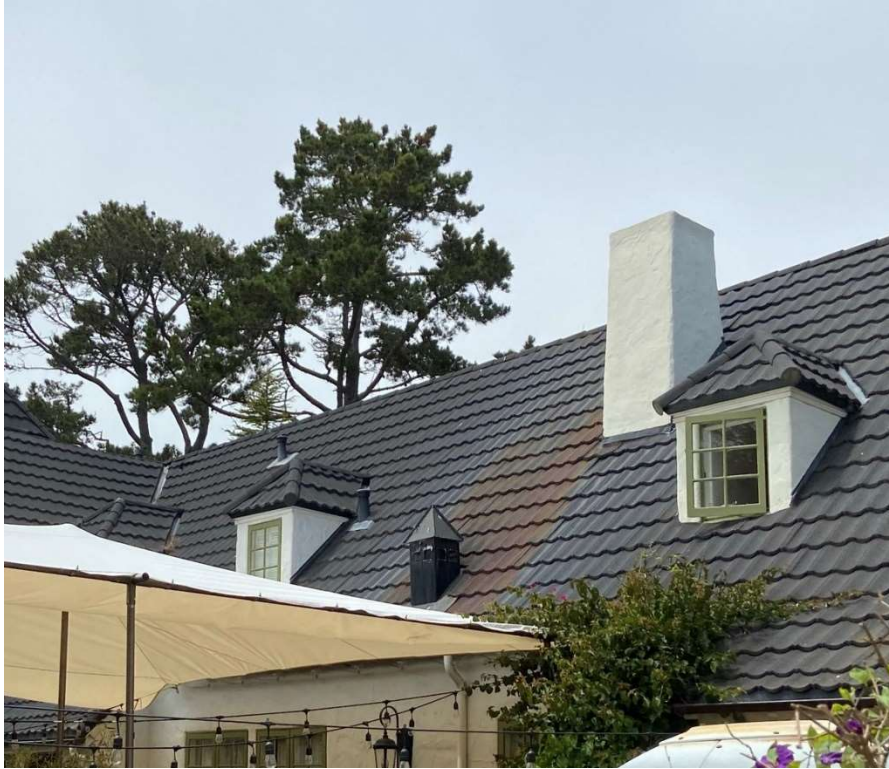
Photo #10, weathered/oxidized roofing at central courtyard
