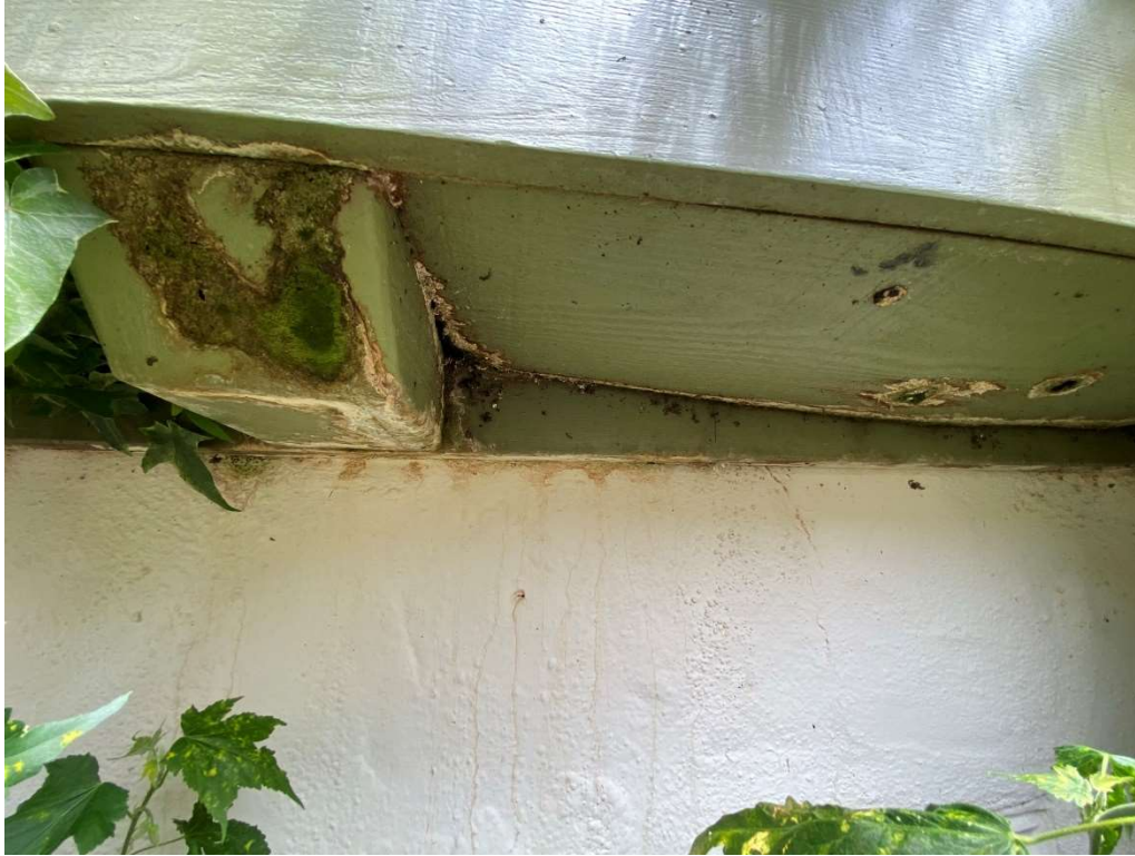
Photo #12, rotted supports at exterior planter box
