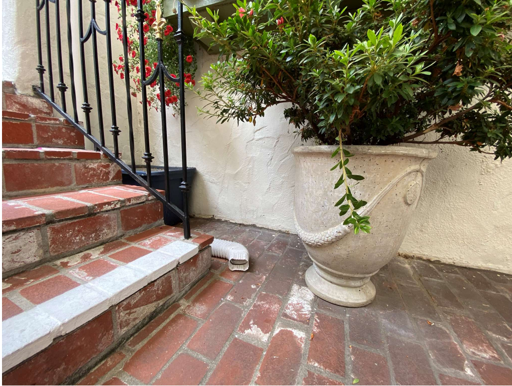
Photo 16, temporary surfact drainage at courtyard
